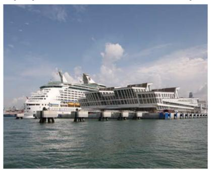
The new cruise terminal consists of two berths and a terminal building. To enable docking by passenger ships on both sides, Penta-Ocean also built a wharf measuring 300 meters long and 120 meters wide and an access deck. The ANDROMEDA V, our large drag suction dredger, was employed to meet the extremely short construction schedule of 27 months.
